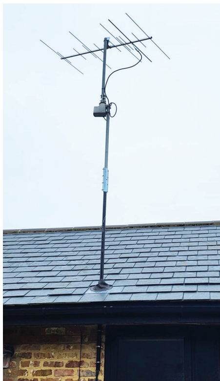
FIGURE 1: The antenna rotator mounted on a pole fixed to my roof.
